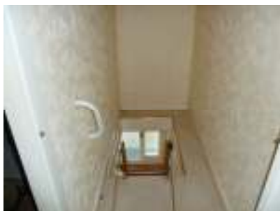
Access by loft ladder to Landing.
