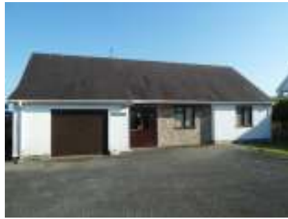
Front Elevation. Excellent drive and turning area.
